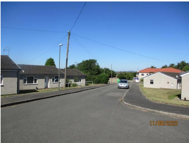
Views within Woburn Close of existing bungalows
