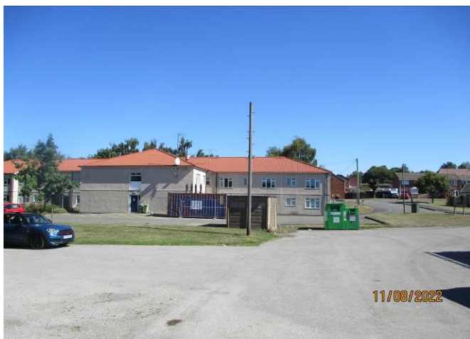
Rear view of Woburn House
