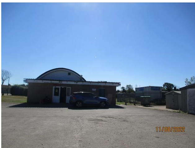
View of existing Community Centre
