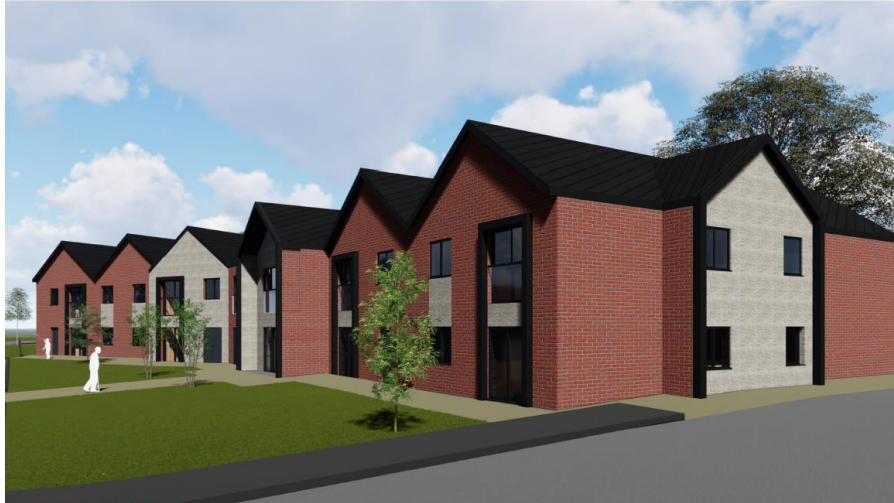
View of Independent Living Scheme Building
